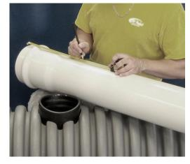
4 Apply an even and smooth coat of certified pipe lubricant to the beveled end of the pipe and to the inside of the FBT.
