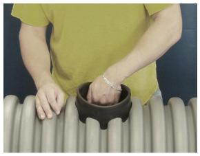
Measure the distance of the FBT from the inside pipe stop to the entrance. Using a belled end or plain end stub of pipe, mark that distance of insertion travel on the leading edge of pipe that will be inserted into the FBT. Cut off the section of the pipe to the desired length. Lightly bevel the leading end of the pipe for easier insertion.
