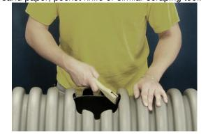
Remove the band clamp from the Fast Branch Tee. Fold and insert it into the drilled opening of the pipe. Unfold the FBT and position it into place and pull up on it until it stops on the inside wall of the pipe.
